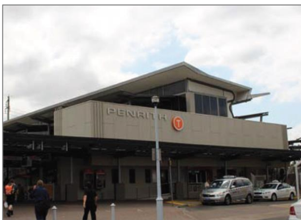
PICTURE 1 – PENRITH STATION TO THE SOUTH OF SITE
