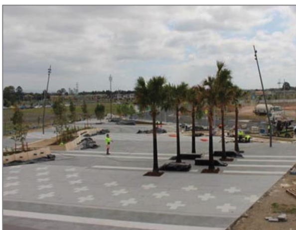
PICTURE 3 – STATION PLAZA ADJACENT TO SITE
